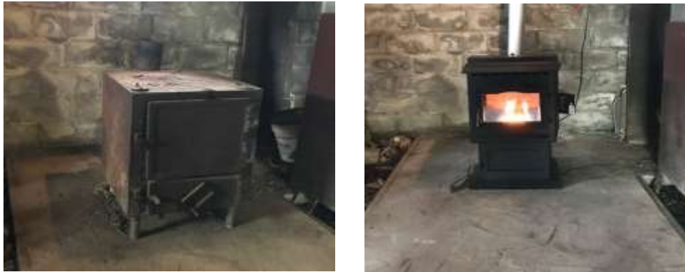
Figure 4. Old wood stove with new wood pellet replacement stove completed by NeighborWorks of Western Vermont
